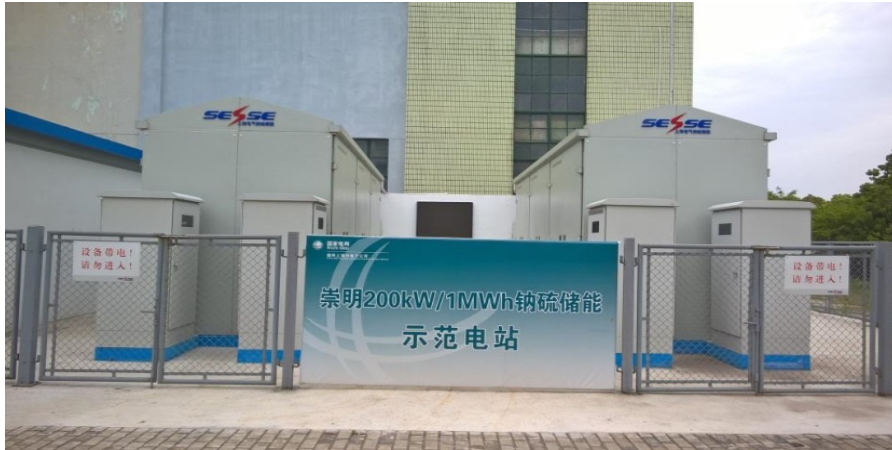
Sodium-sulfur BESS Station
